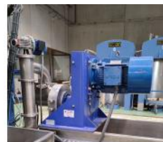
Reference: MZA-012 CRUSHER MILL Year: 2004 Brand: ALFA LAVAL
